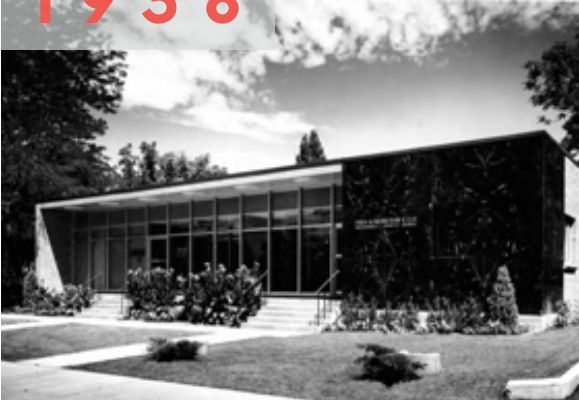
THE FRED A. MORETON & COMPANY BUILDING
